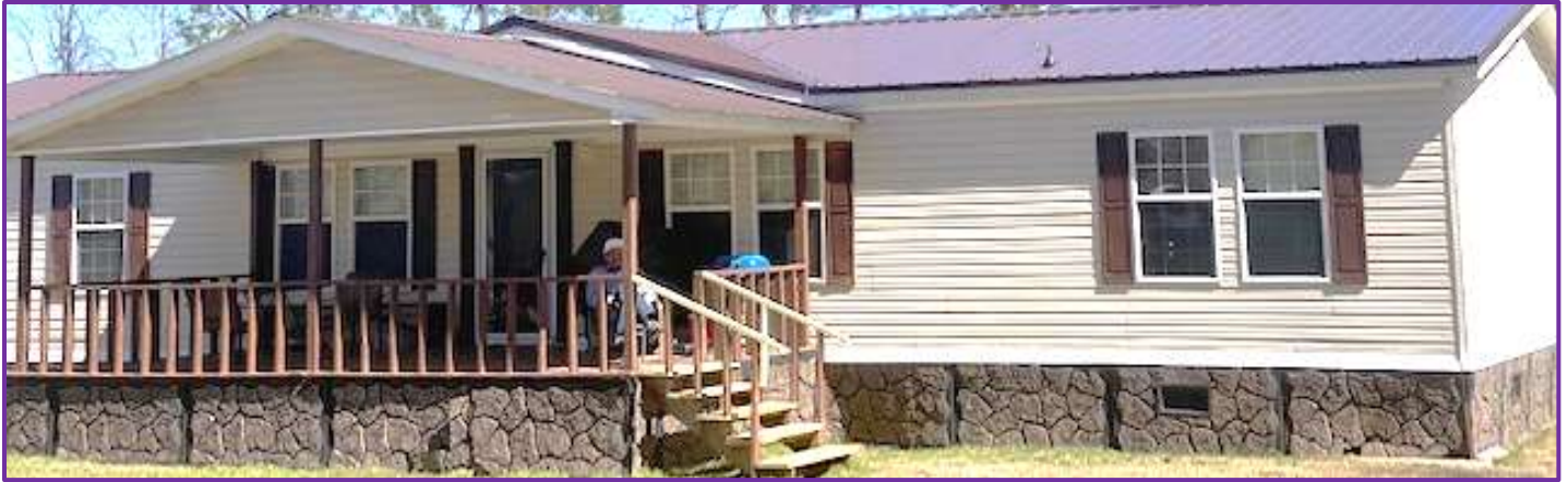
Roosevelt Woodley, a satisfied client, enjoys a bright sunny day on his front porch after a new roof and other needed repairs have been made to his home through the CSLC Federal Home Loan Bank of Dallas/BankPlus Affordable Housing Rehabilitation Program.
